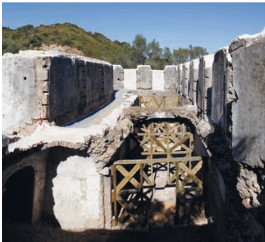
Structural stabilization of pre-existent walls: connecting elements of wooden parts (reversible), 2011
