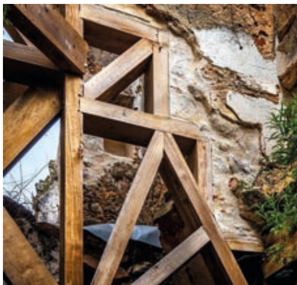
Structural stabilization of pre-existent walls: connecting elements of wooden parts (reversible), 2011
